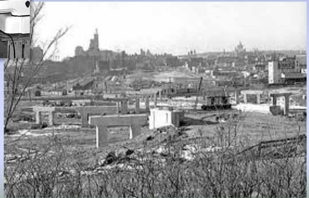
I94 construction St. Paul MN
